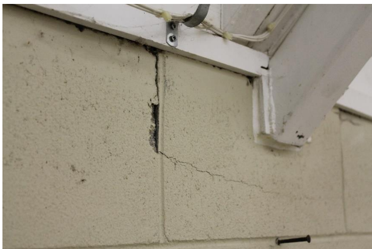
Earthquake Damage Critical Structure weakness – squash court
