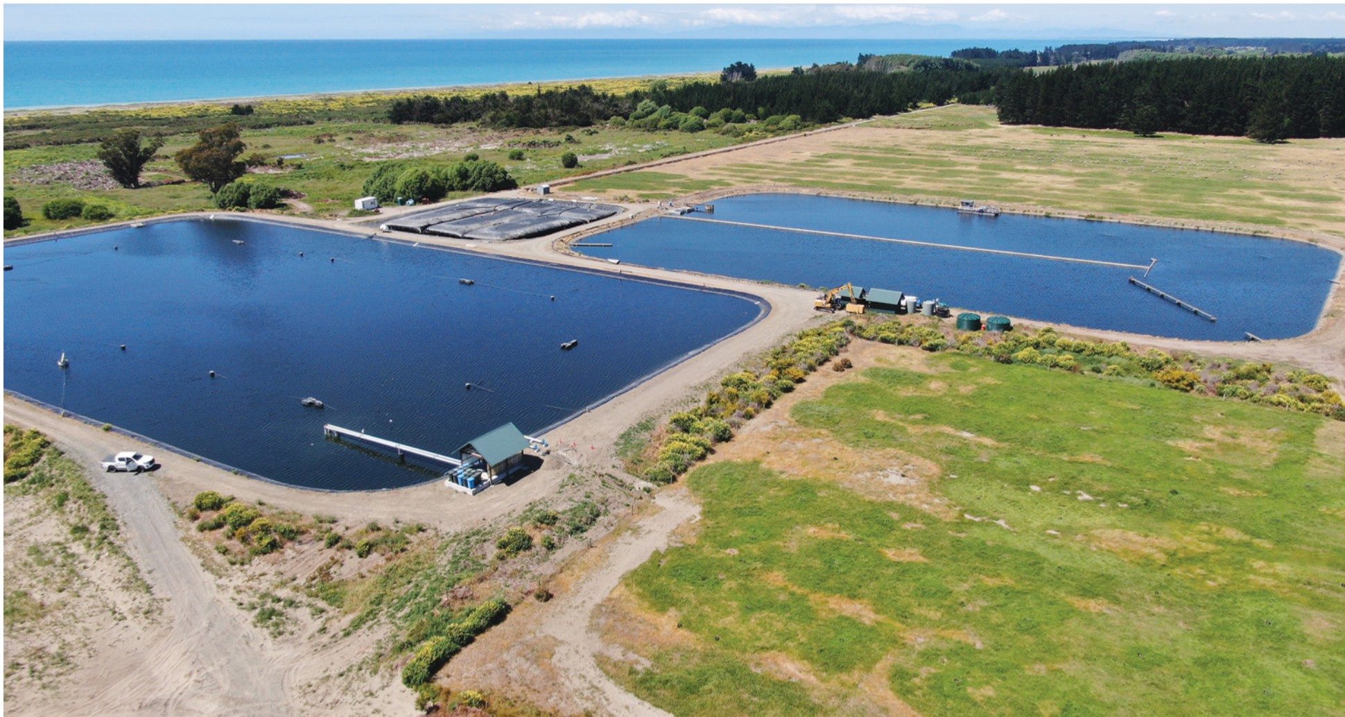
The work has included adding a new wet-well for the collection of the treated water, and a new treatment shed for better control and monitoring of the irrigation systems in place.
