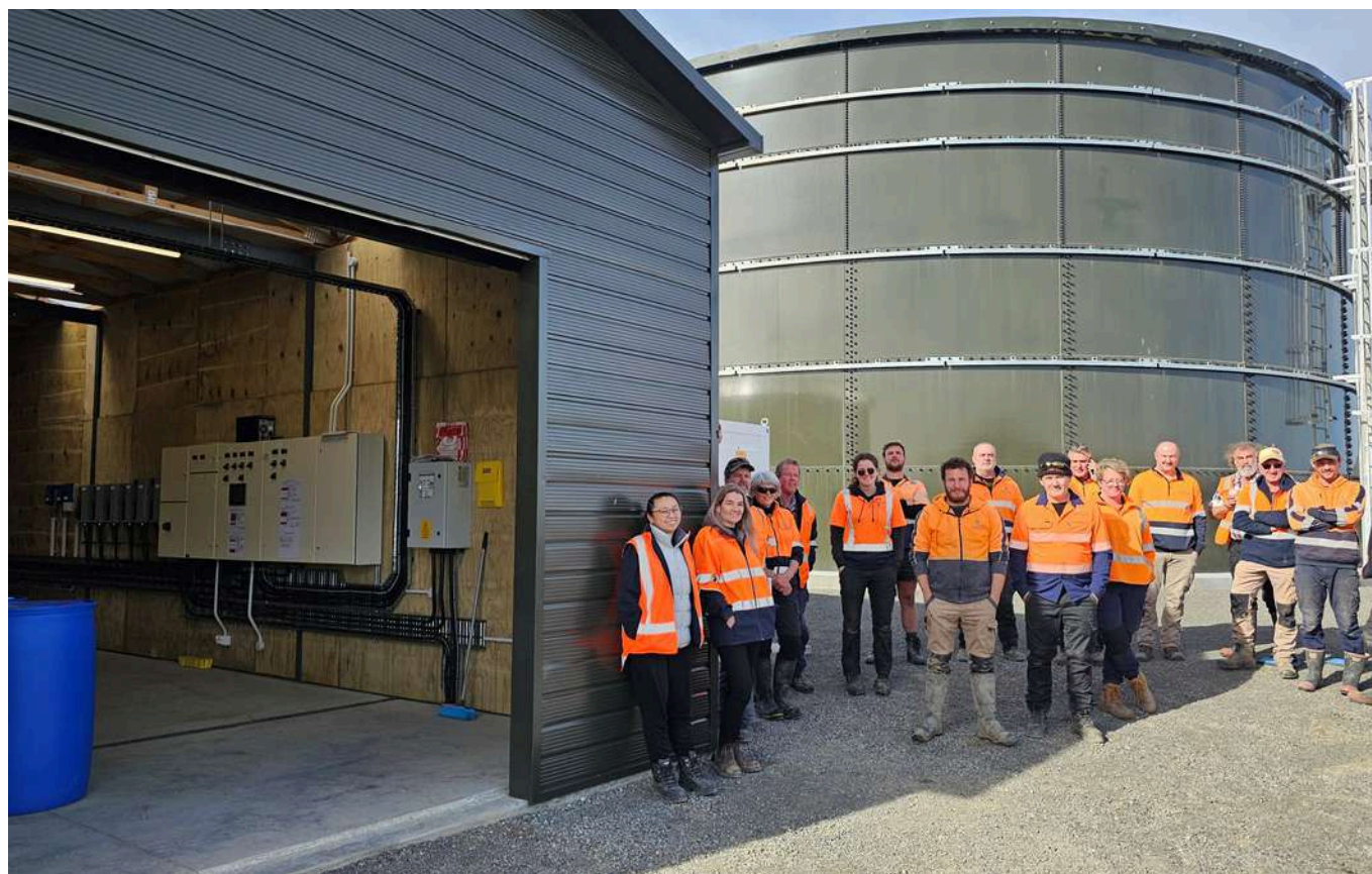
The new reservoir at the Bishells water treatment plant has increased the scheme’s resilience. It is now possible to shutdown the plant for repairs and maintenance without impacting water supply to customers.
