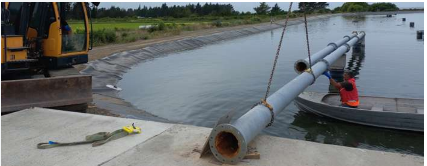
Replacement of the intake at the Amberley sewerage plant
