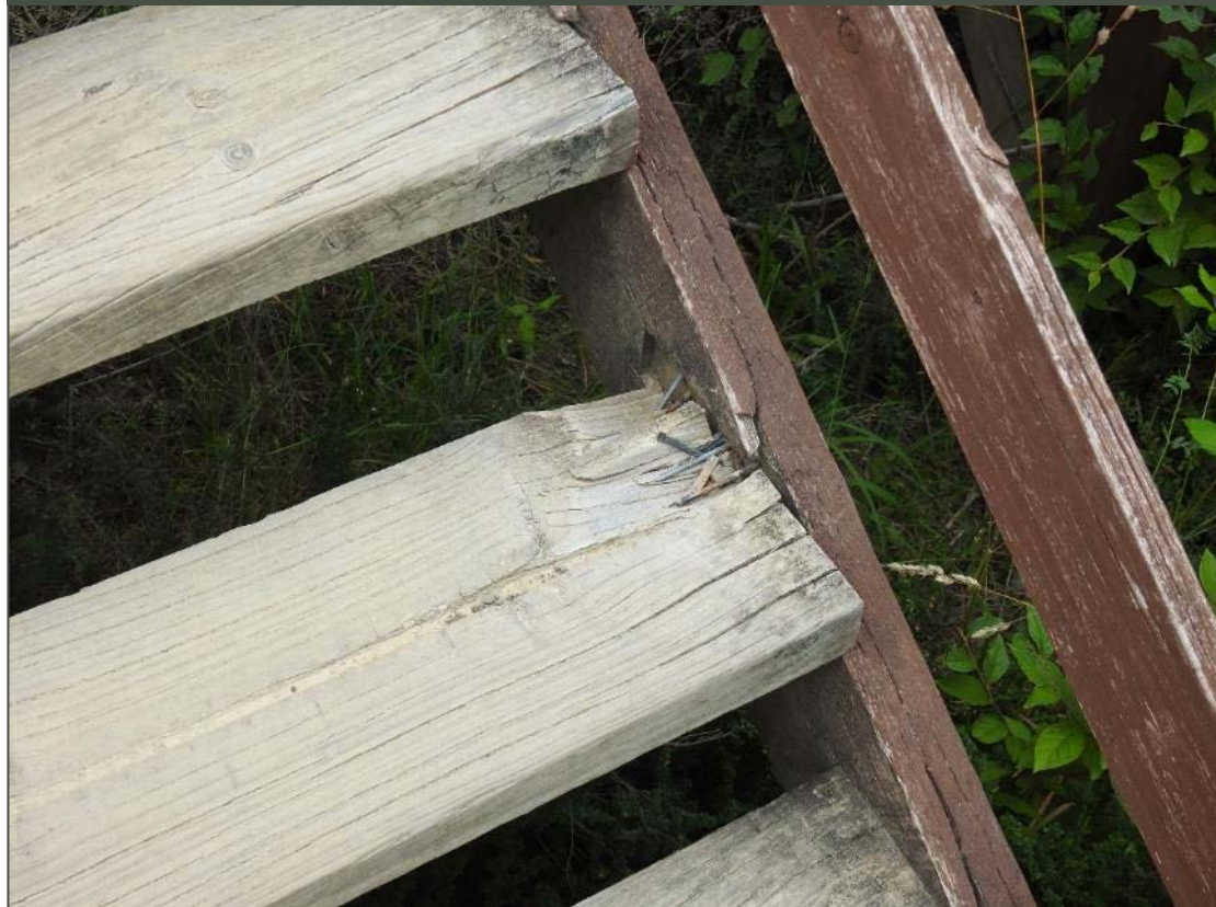
Figure 6: Conical Hill facility condition example
